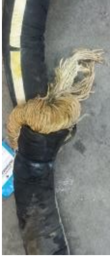
EXPOSED CUT FIBRES
